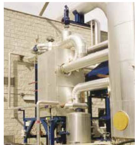
AlfaVap thermosiphon reboiler at Carboneco in Spain. The AlfaVap is used to boil 30% MEA at the bottom of the stripping column. The absorption-stripping system at Carboneco is used to recover carbon dioxide from a cogeneration plant. The system was built by the Danish contractor Union Engineering.
